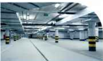
ENCLOSED CAR PARK
