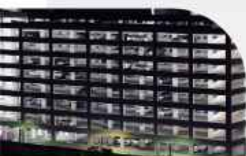
OPEN CAR PARK
